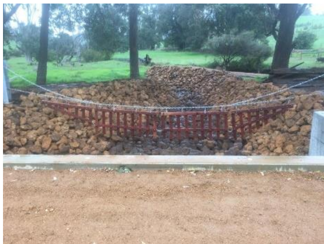
Lyons Road Bridge Replacement
