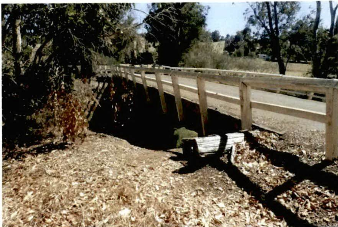
Photo No. 2: Left hand side view from abutment 1. (Taken: 24-Jan-2018)
