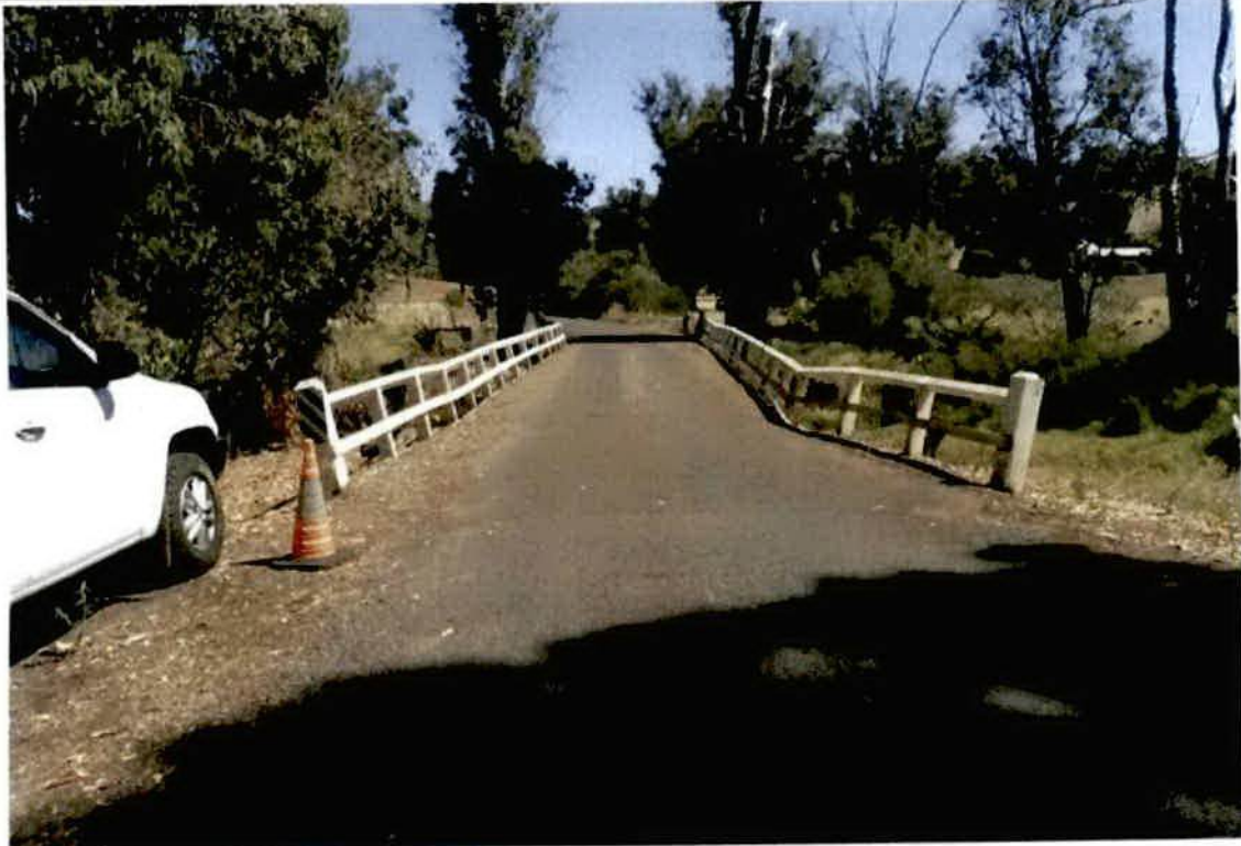
Photo No. 1: Overall view from abutment 1. (Taken: 24-Jan-2018)
