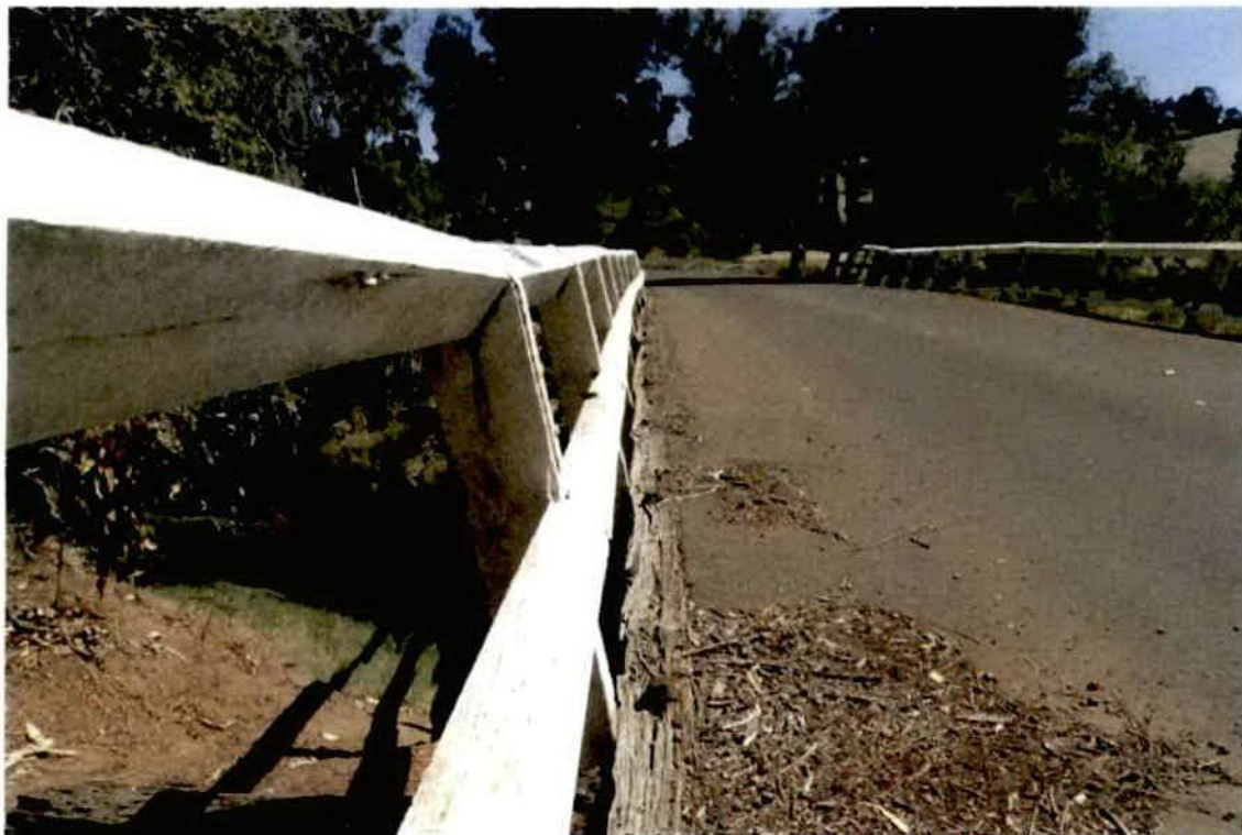
Photo No. 12: Left hand side v-barrier at abutment 1 end. (Taken: 24-Jan-2018)
