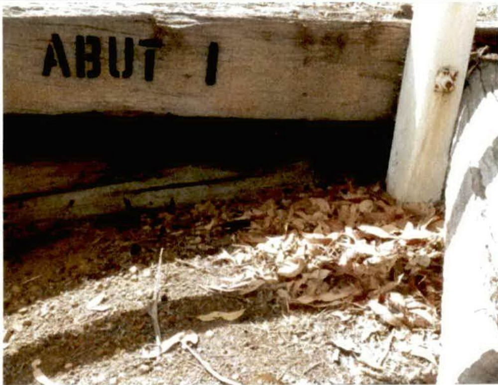
Audit Photo No. 1: Span 1 LHS, deck ends U/S. (Taken: 15-Mar-2018)
