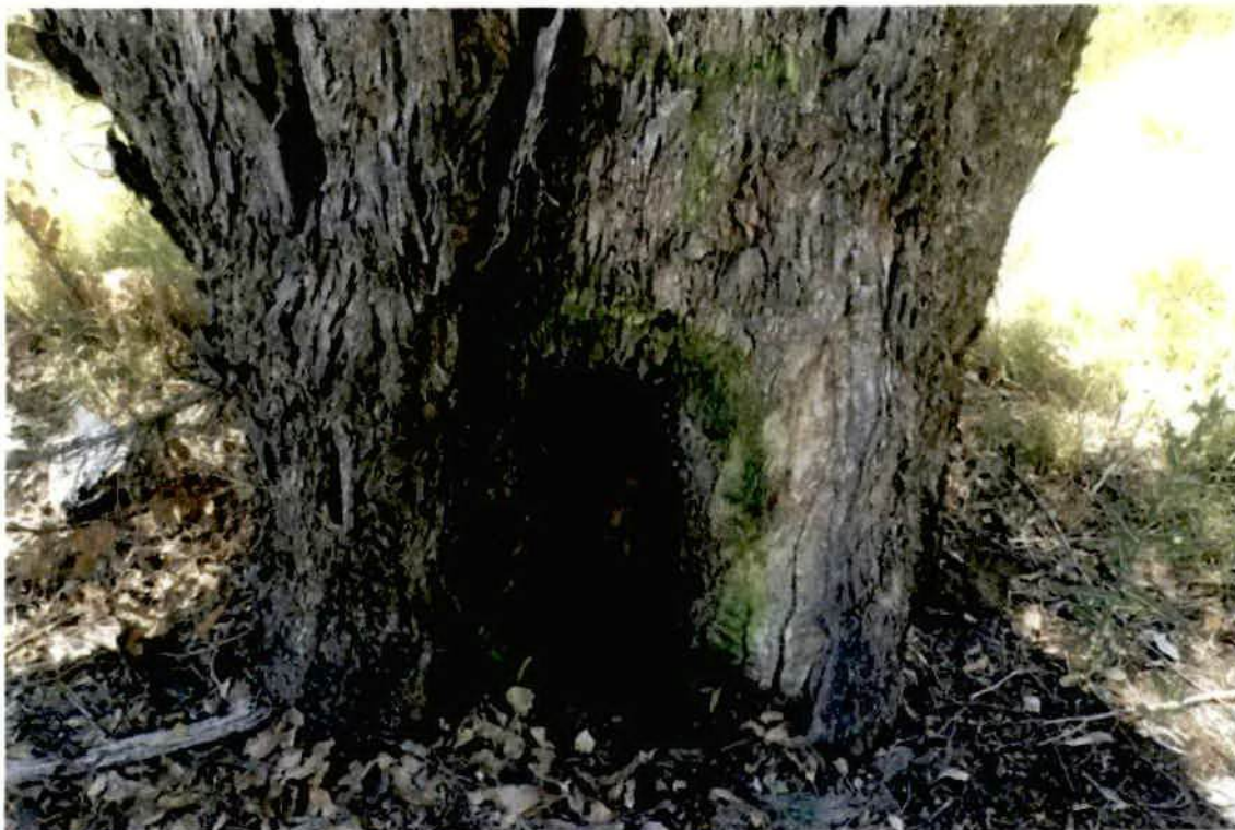
Photo No. 20: Termite nest in base of tree at abutment 2 right hand side, at barrier termination. (Taken: 24-Jan-2018)
