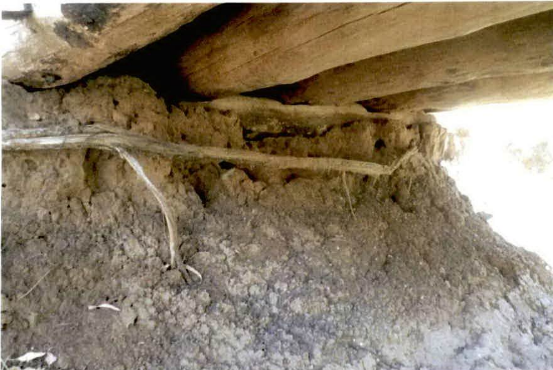
Photo No. 8: Abutment 2 face from left hand side. (Taken: 24-Jan-2018)
