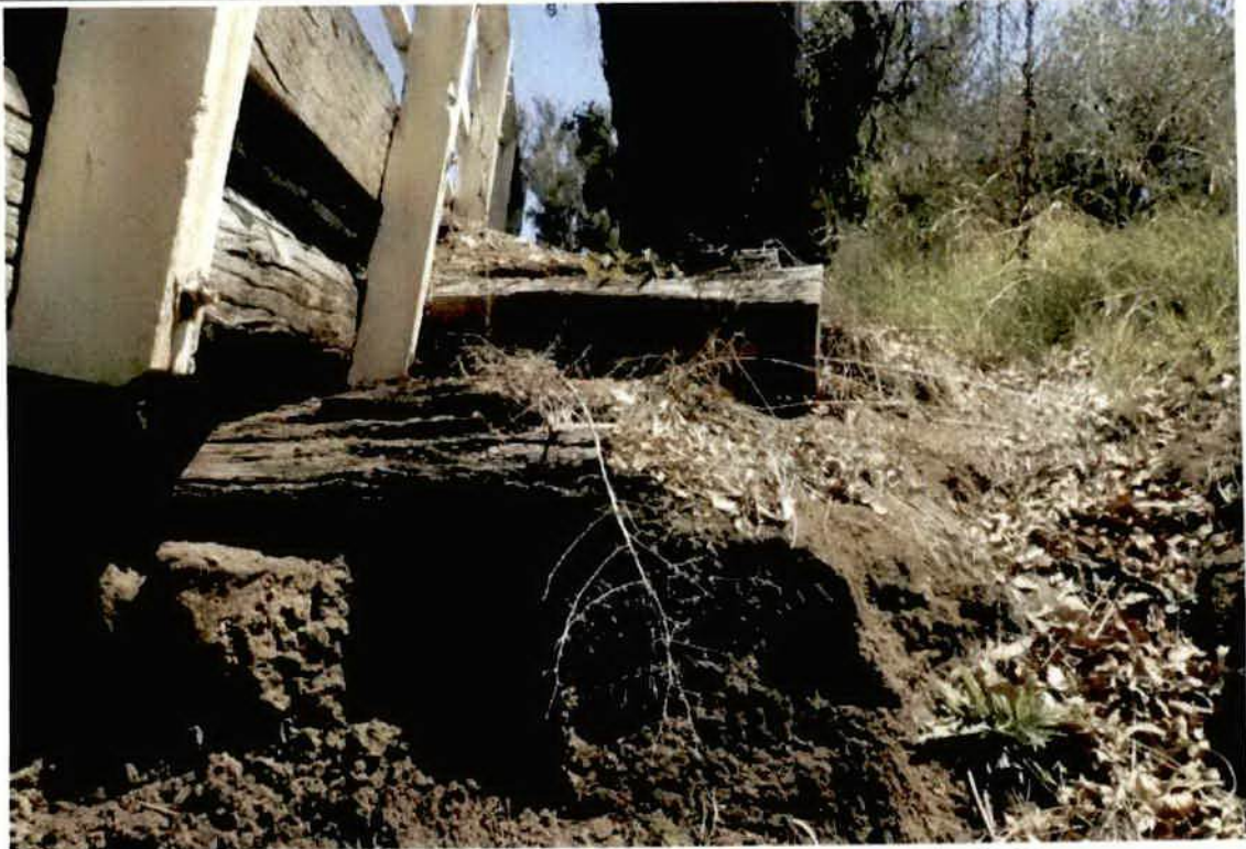
Photo No. 9: Right hand side wingwall at abutment 2. (Taken: 24-Jan-2018)
