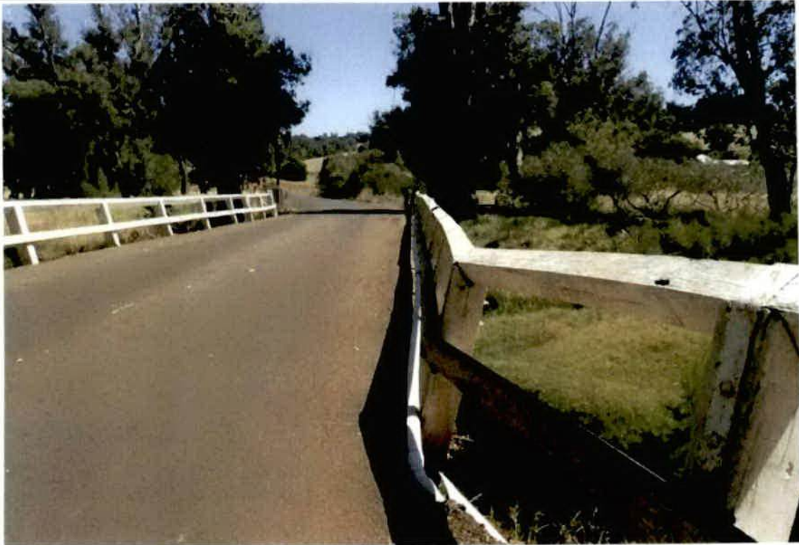
Photo No. 13: Right hand side v-barrier at abutment 1 end. (Taken: 24-Jan-2018)
