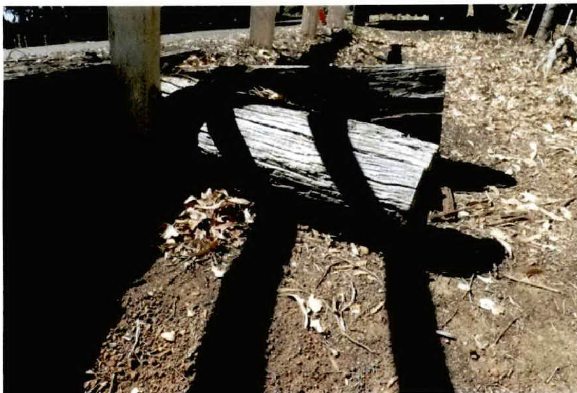
Photo No. 4: Left hand side wingwall at abutment 1. (Taken: 24-Jan-2018)
