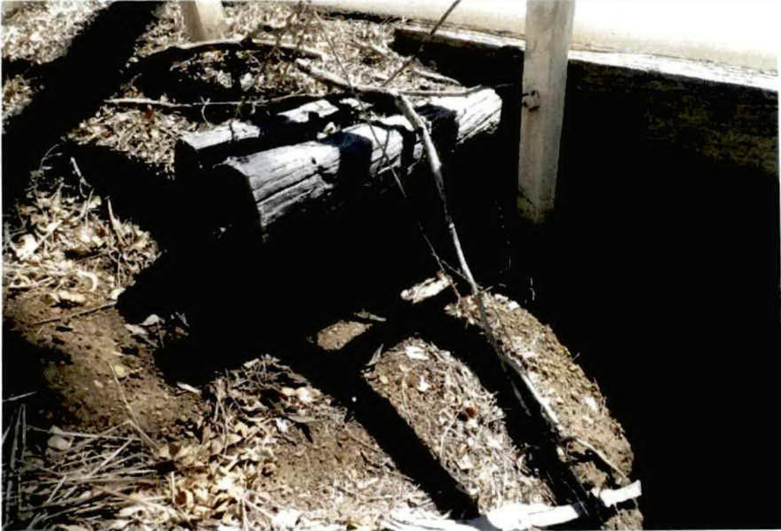
Photo No. 7: Left hand side wingwall at abutment 2. (Taken: 24-Jan-2018)
