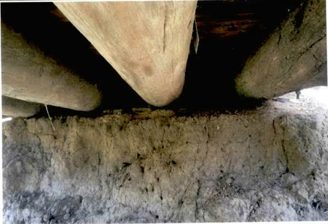
Photo No. 5: Abutment 1 face from left hand side. (Taken: 24-Jan-2018)
