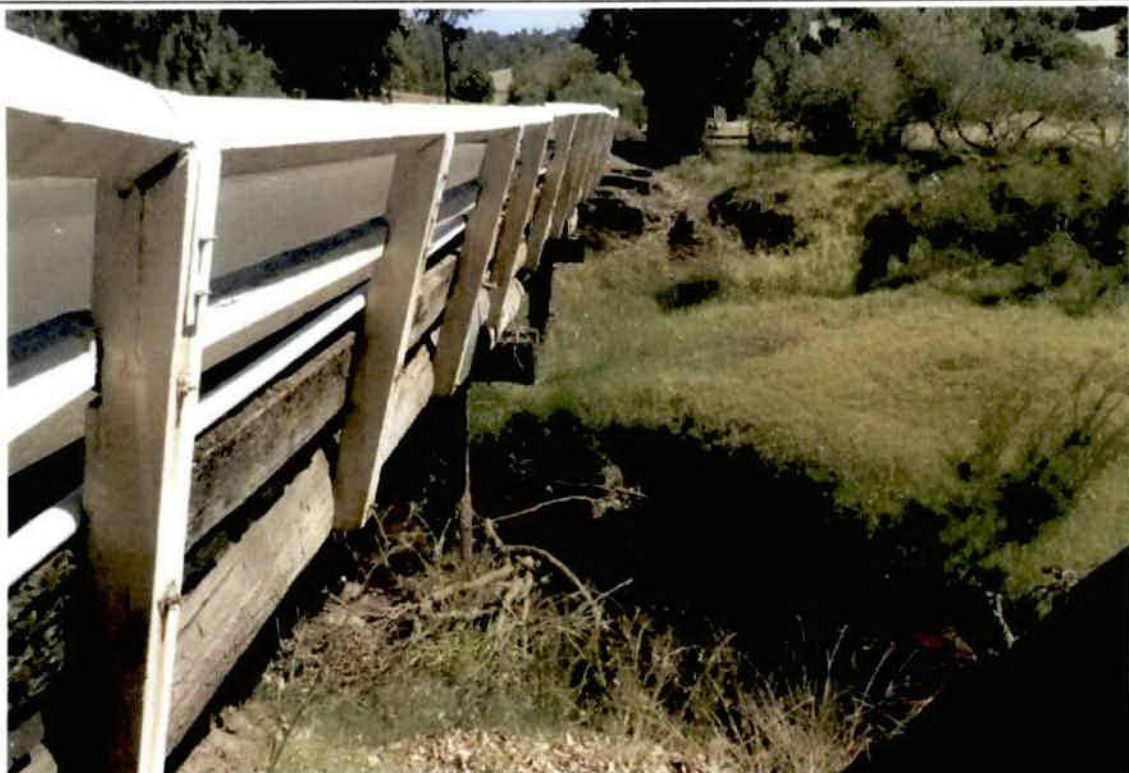
Photo No. 15: Right hand side v-barrier from abutment 1 wingwall. (Taken: 24-Jan-2018)
