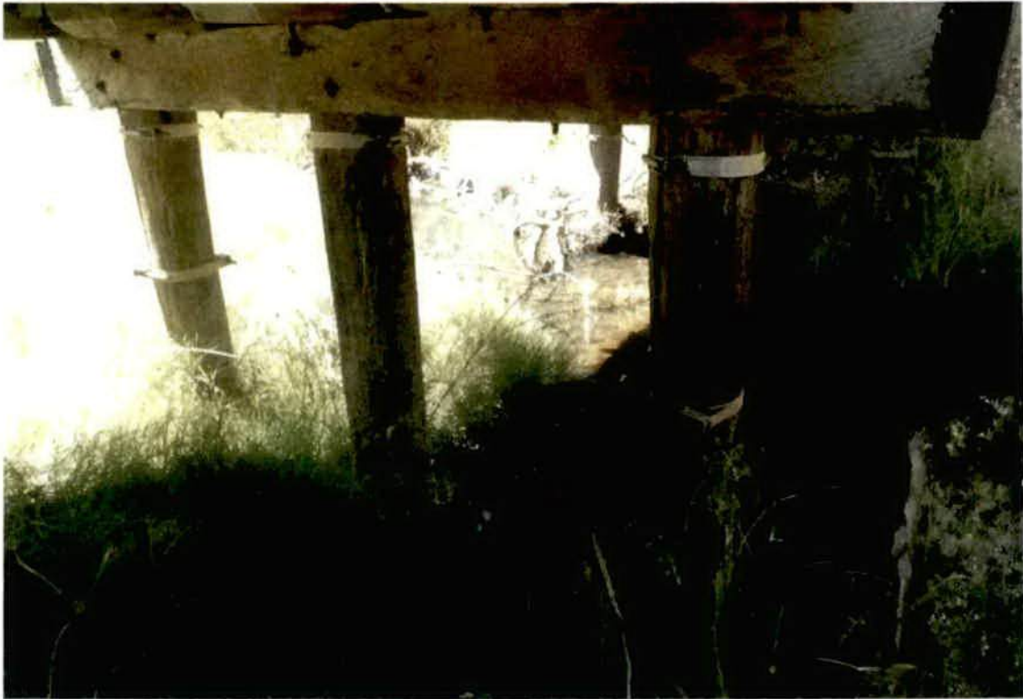
Photo No. 11: Pier 2 layout from left hand side. (Taken: 24-Jan-2018)
