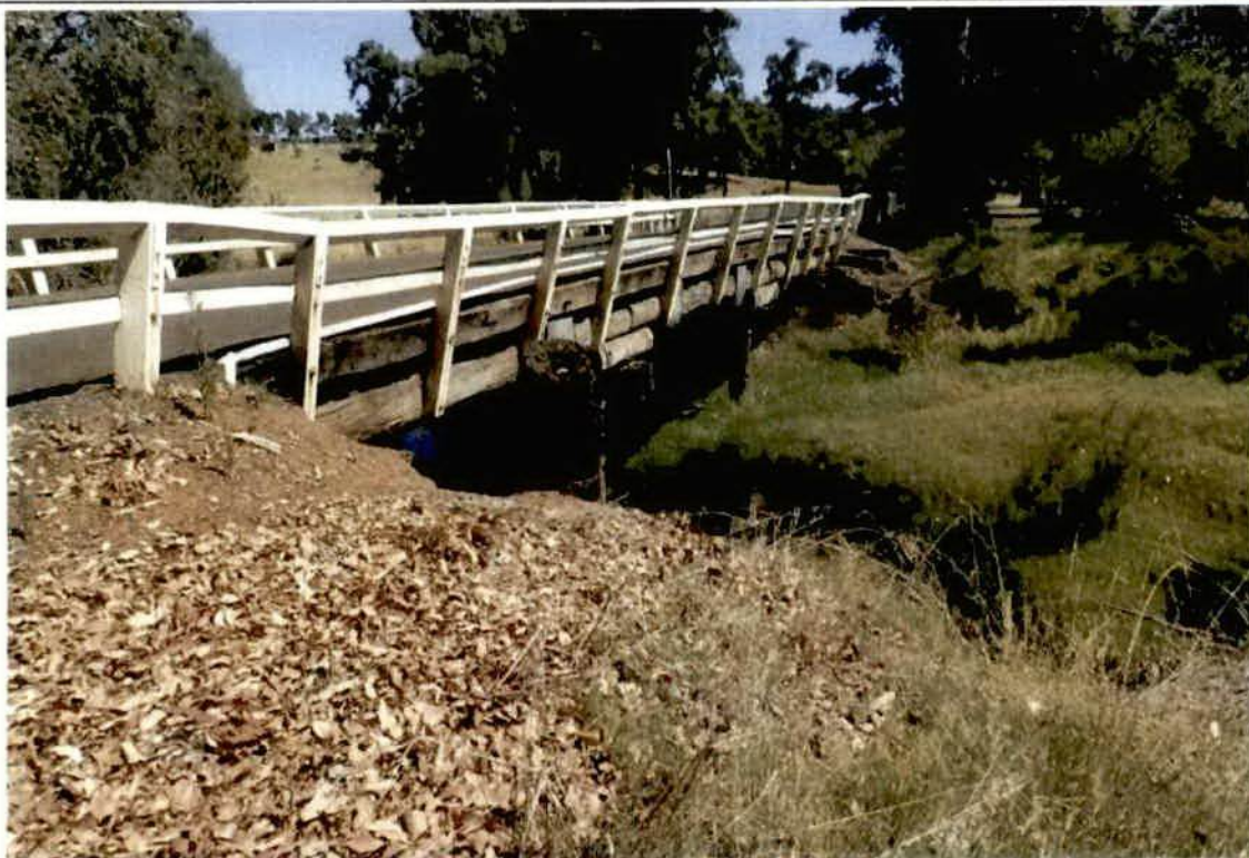
Photo No. 3: Right hand side view from abutment 1. (Taken: 24-Jan-2018)
