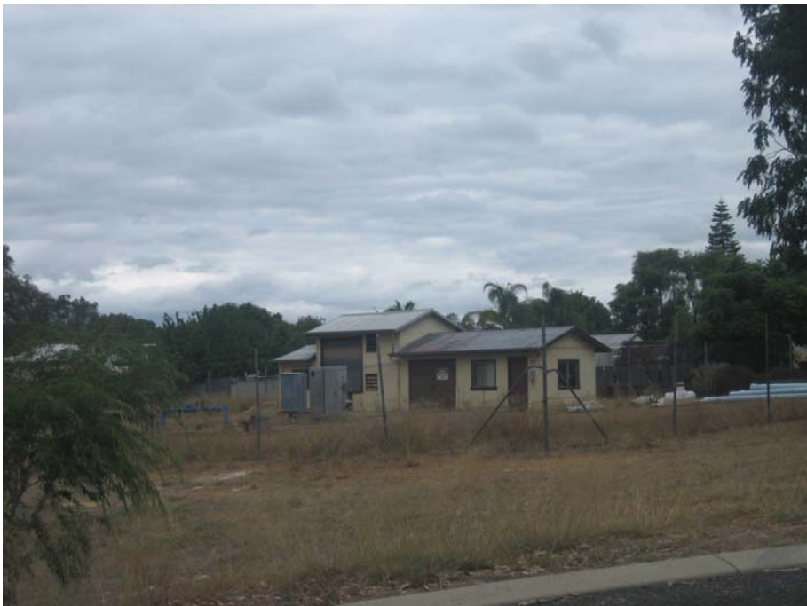
Figure C2 Production bores 1/75 and 2/82
